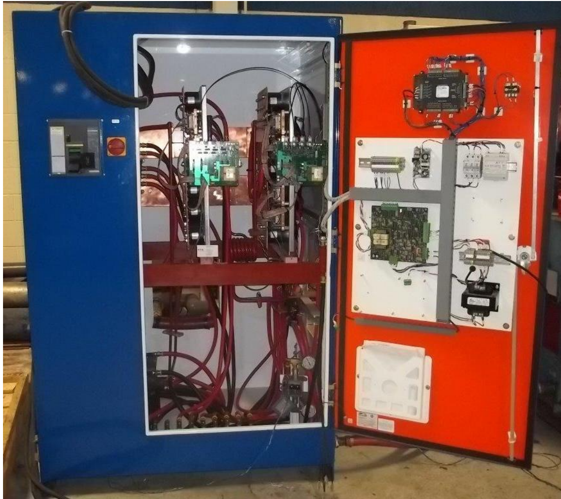
Interpower Induction controller being built up
